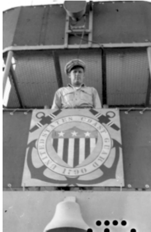
Lt. Adams on bridge remodeled by Navy Seabees
