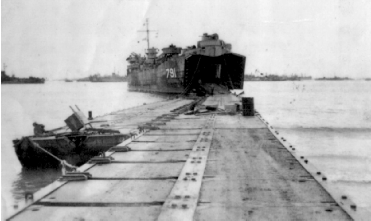
Unloading ammunition using pontoons at Okinawa
